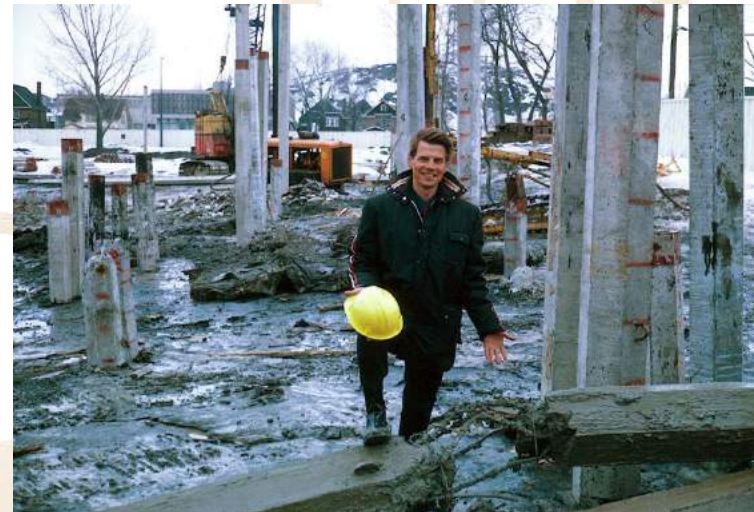
1974 Timmins, Ontario, resolving cause of broken piles
