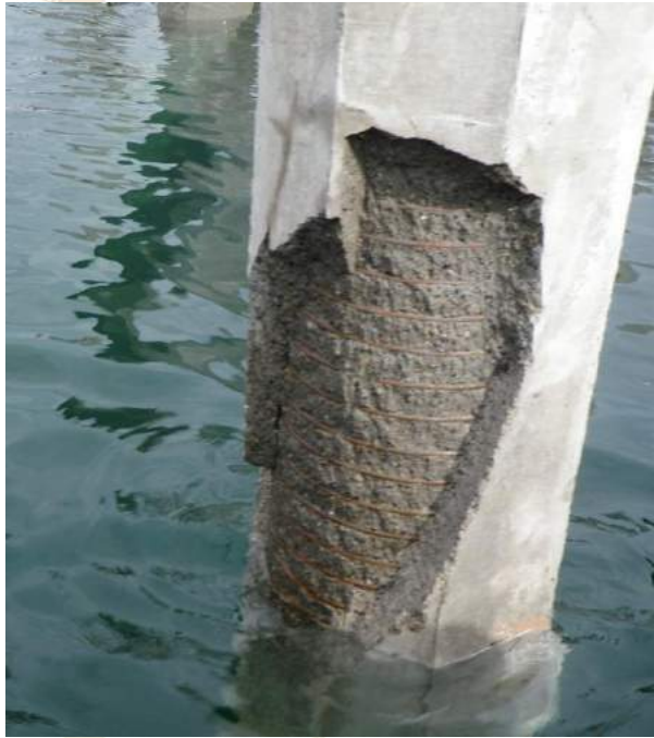
Too thick cover on hard driven piles
