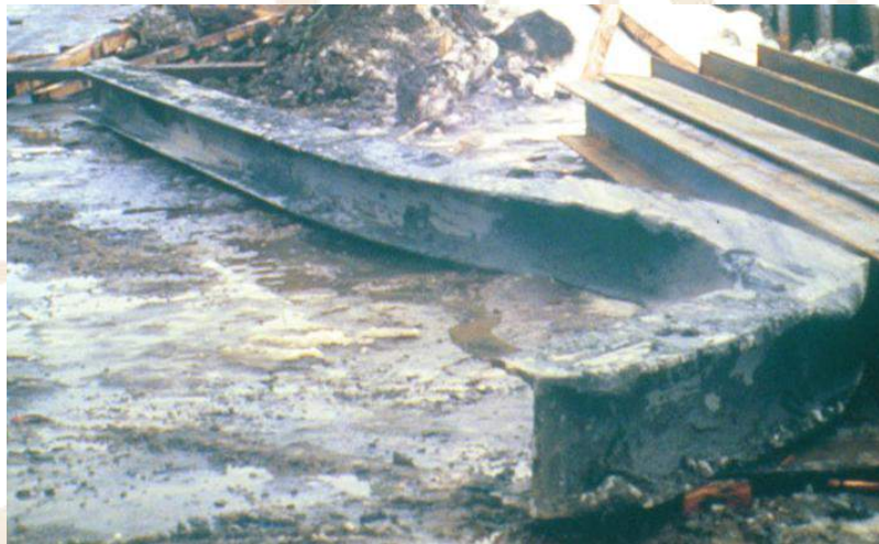
H-pile driven to sloping bedrock
