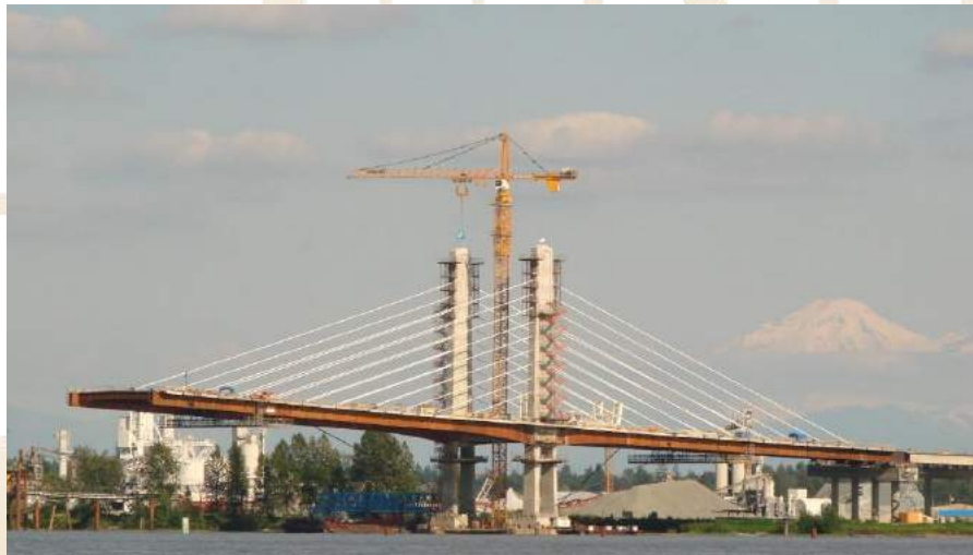
2008 Golden Ears Bridge, Vancouver, BC. “Pile pad” on floating piles in marine clay.
