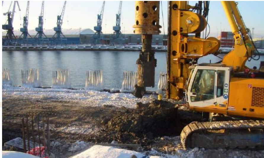
2006 Harbor in Muuga, Estonia. Settlement of 45 m long pipe piles
