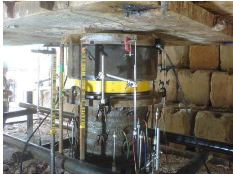
2007 Orchard Center, Singapore. Head-down and bidirectional test on same pile
