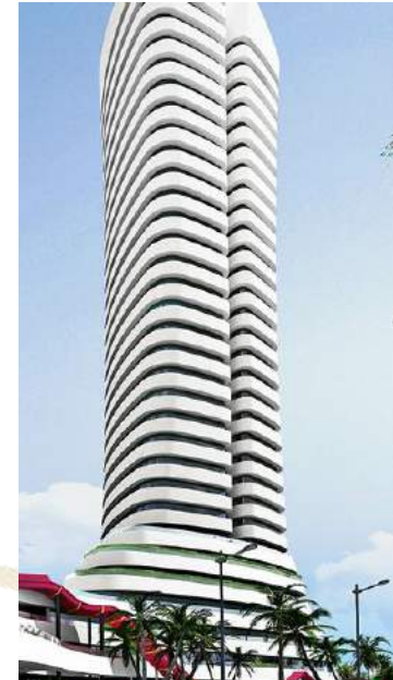
2008 Amwaj Tower, Dubai. Evaluation of full-scale multi-level bidirectional loading tests.
