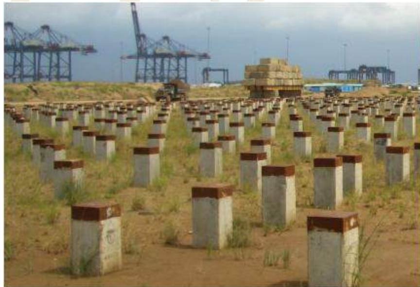
2011 Cai Mep Container Port, Vietnam. Remediation of excessive settlement after a failed wick drain treatment.
