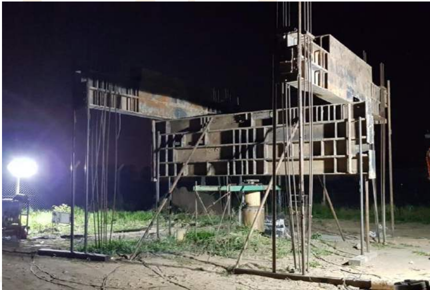
Ready for one of 25 loading tests.
