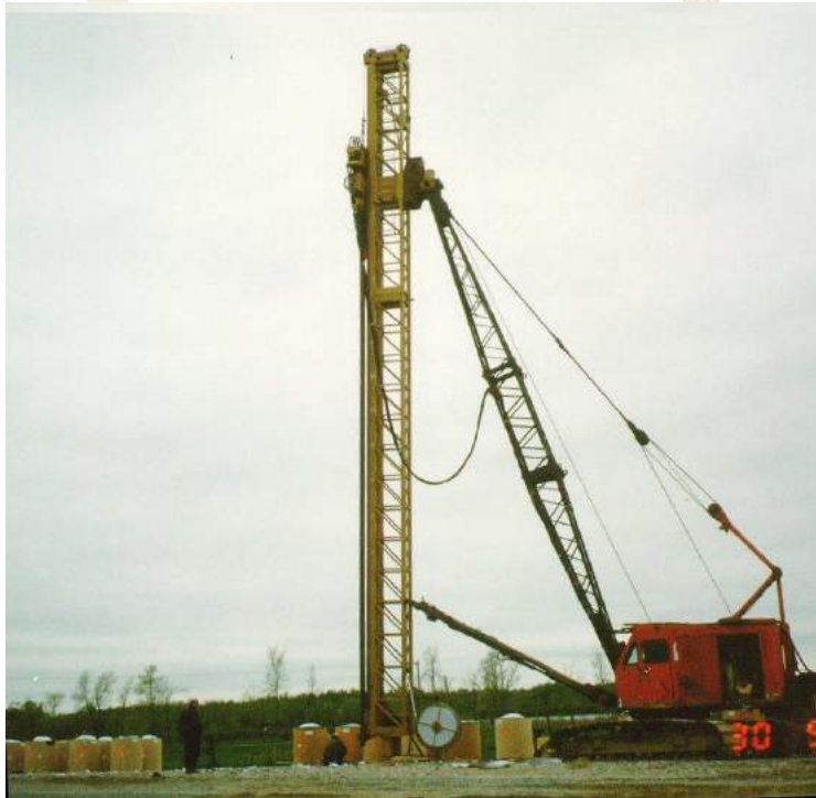
2000 HWY416, Ontario, wickdrain full-scale project
